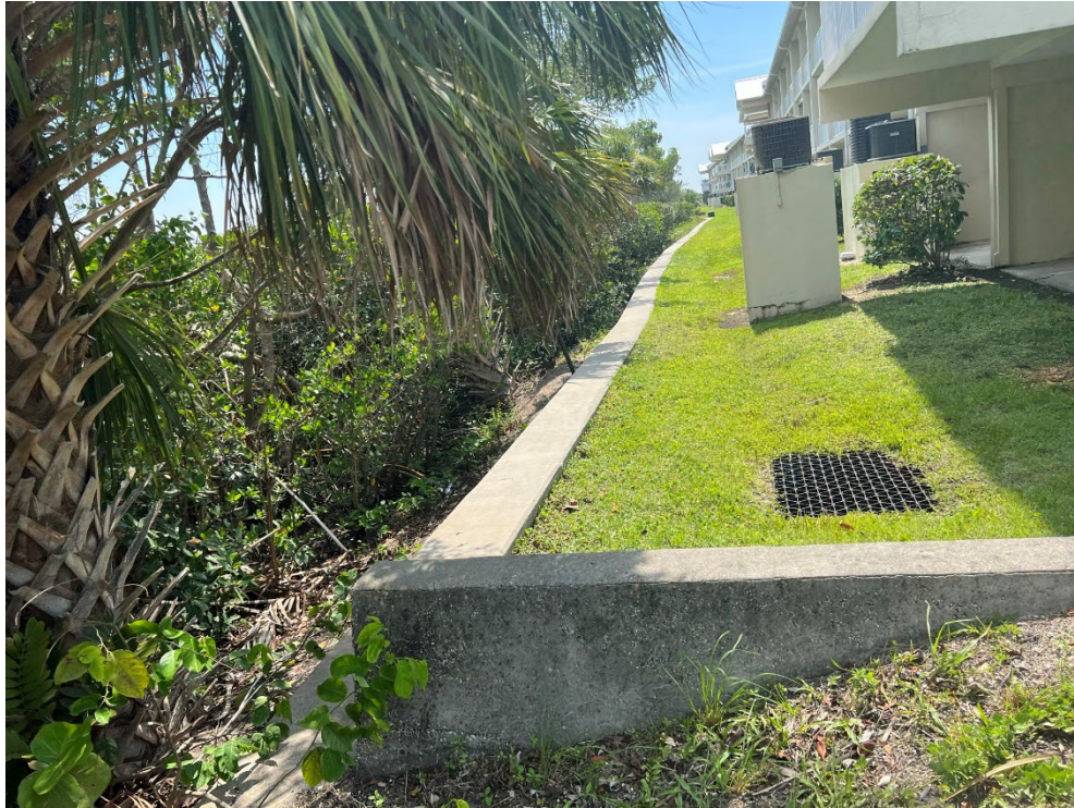
Photo #8 – Top View of the Wall Near the End of Section 1.
