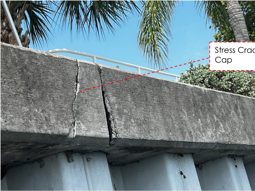
Photo #3 – Stress Cracking in the Cap.
