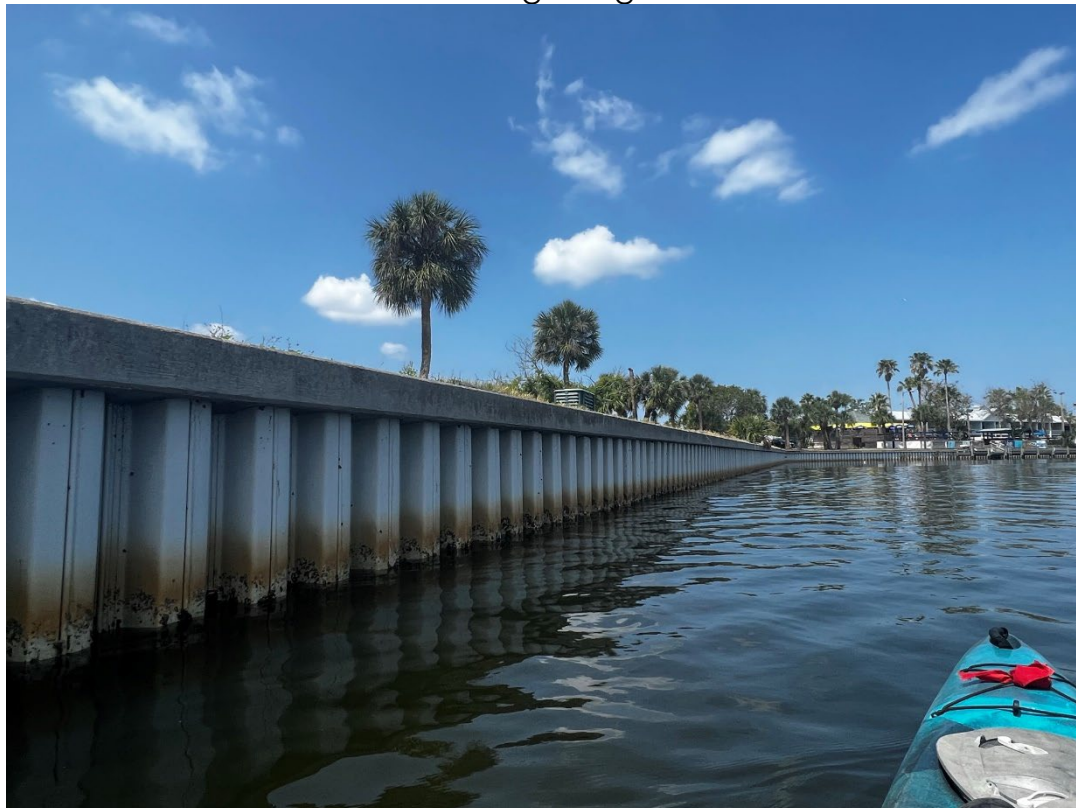
Photo #1- East End of Seawall. Beginning of Section 2.
