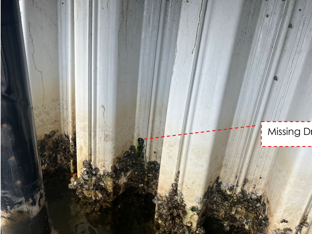
Photo #5 – Missing Drain.
