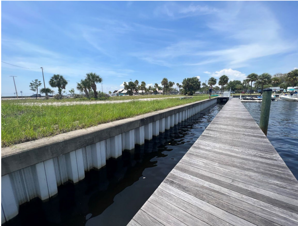
Photo #4 – Front View of the Seawall.
